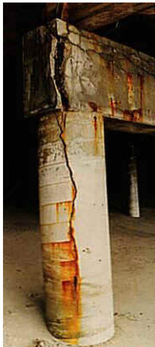
Fracture of concrete
