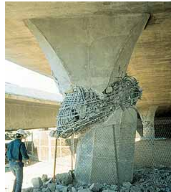
Failure of column
