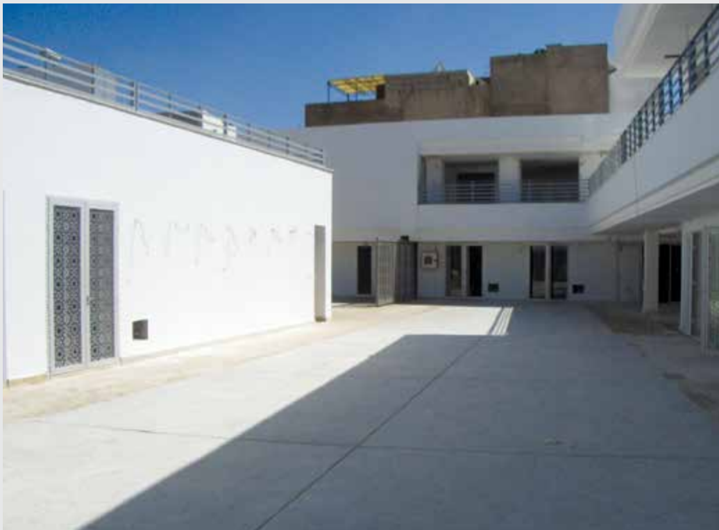
New Foundouk for artisanal subcontractors at Ain Nokbi (internal view)
