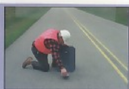
3. The Protect Cover and Counter are retrieved after the traffic study is completed and the Protective Cover can be used for the next installation.
