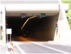
Branisko Tunnel, Slovak Republic
