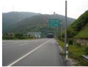
Tianpingling Tunnel, China
