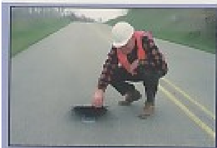
1. The Protective Cover is placed over the Counter in the center of the traffic lane.
