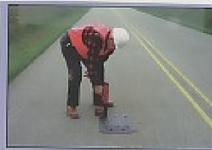
2. The Protective Cover is fastened to the roadway using a powder-actuated nail gun.
