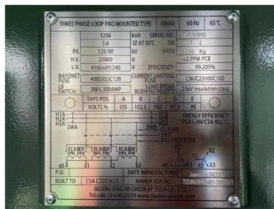
Figure 3. Plaque signalétique d'un transformateur triphasé 1250 kVA. Source <https://daelim-electric.com/wp-content/uploads/2022/10/transformer-nameplate1-1536x1152.webp>
