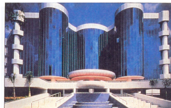
FIGURE 2. Glazing on a building may be the most important component of the building's exterior aesthetic quality, which leads to thin-film glass-coating effects on incident light.
