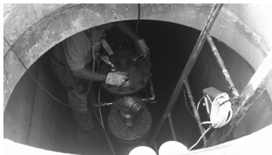
Figure 4: This photo shows a VOMWD employee manually changing the PRV setting.
