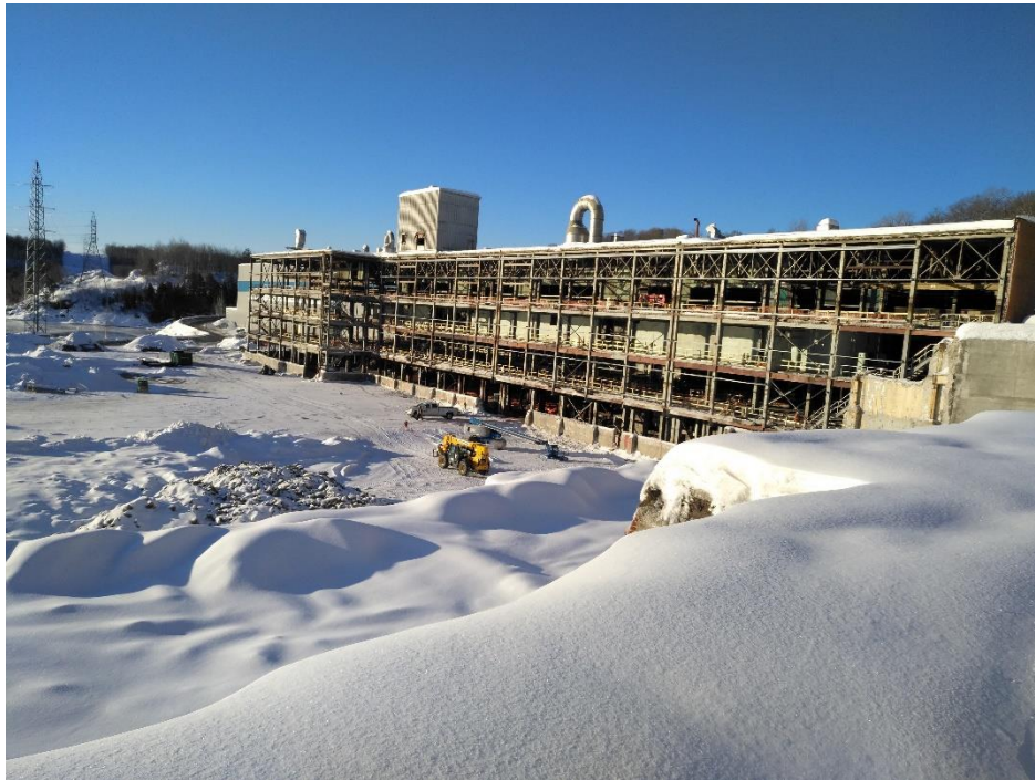
Figure 24.18 – Building #67 East Wall Cladding and Structural Reinforcement
