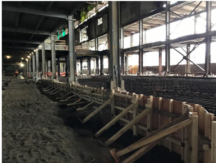
Figure 24.20 – Building 67 Formwork & Rebar for Pile Caps and Tank Foundations
