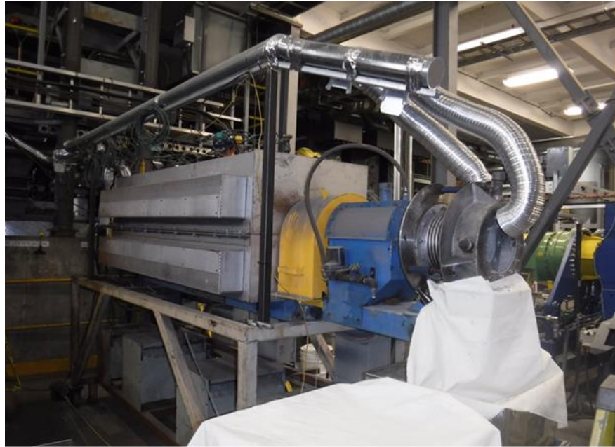
Figure 13.15 – Pilot Acid Bake Kiln at COREM
