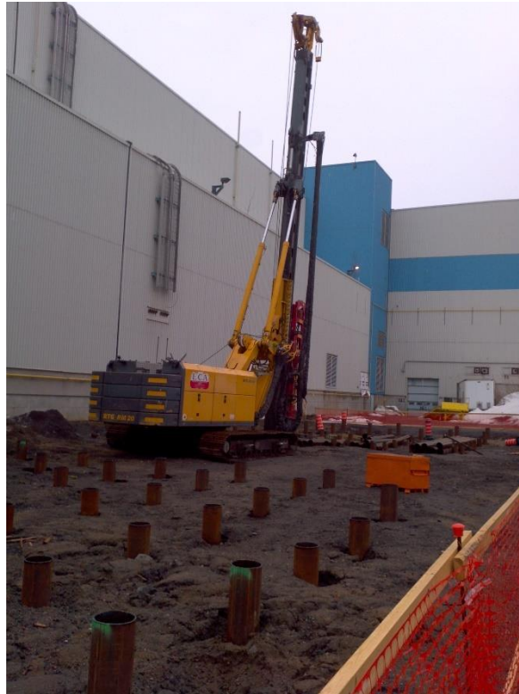
Figure 24.21 – Piling West of Building #80
