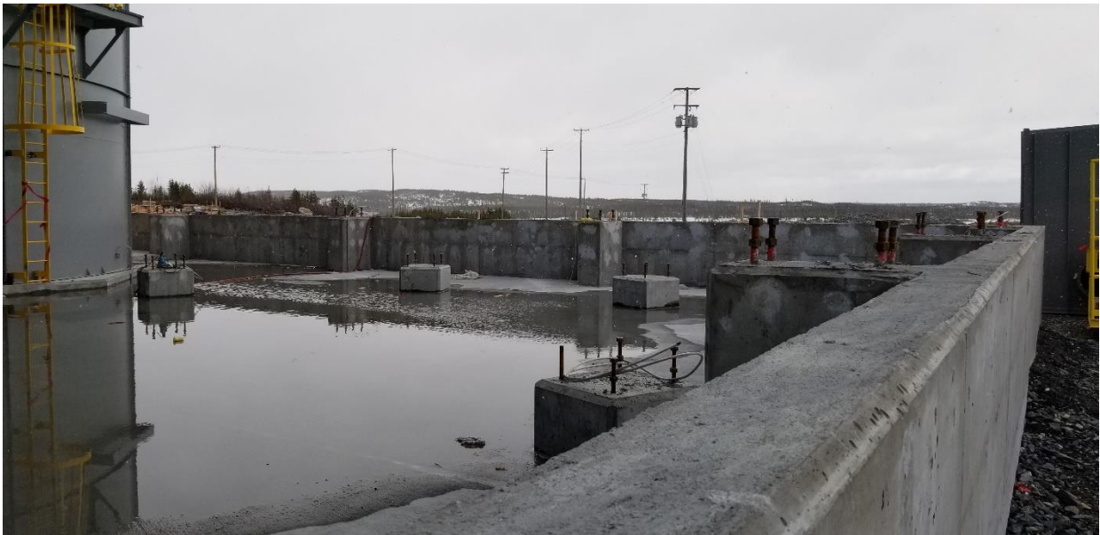
Figure 24.9 – View of the Process Water Tank and Thickener Area
