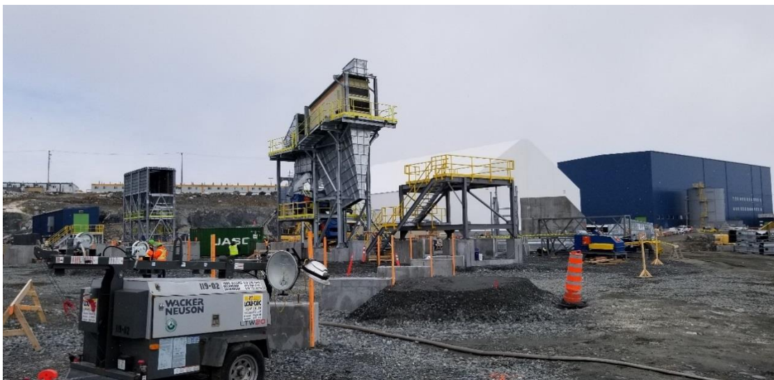
Figure 24.4 – View of Screening Tower, and Concentrator
