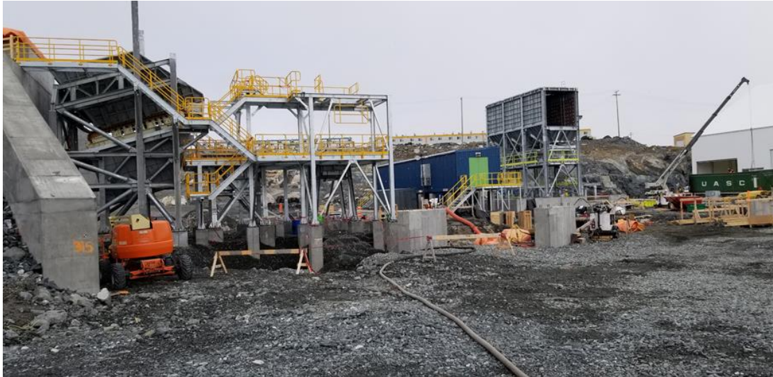
Figure 24.3 – View of Primary and Cone Crusher Buildings
