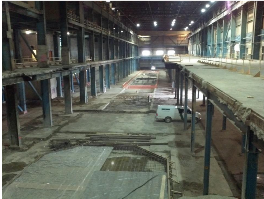
Figure 24.19 – Building #80 Form Work and Rebar for Tanks Foundations
