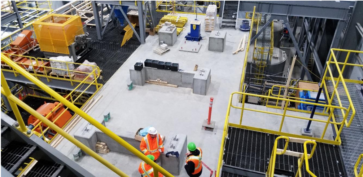
Figure 24.10 – View of the Dryer Foundations
