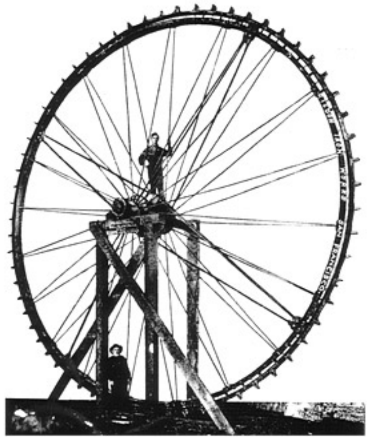
30 foot water wheel with Risdon cups, North Star Power House, Grass Valley, CA, 1895.
