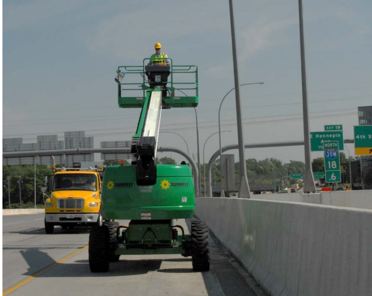
Figure 17. I-35W luminaire cleaning, showing MNDOT lane closure and man lift used.
