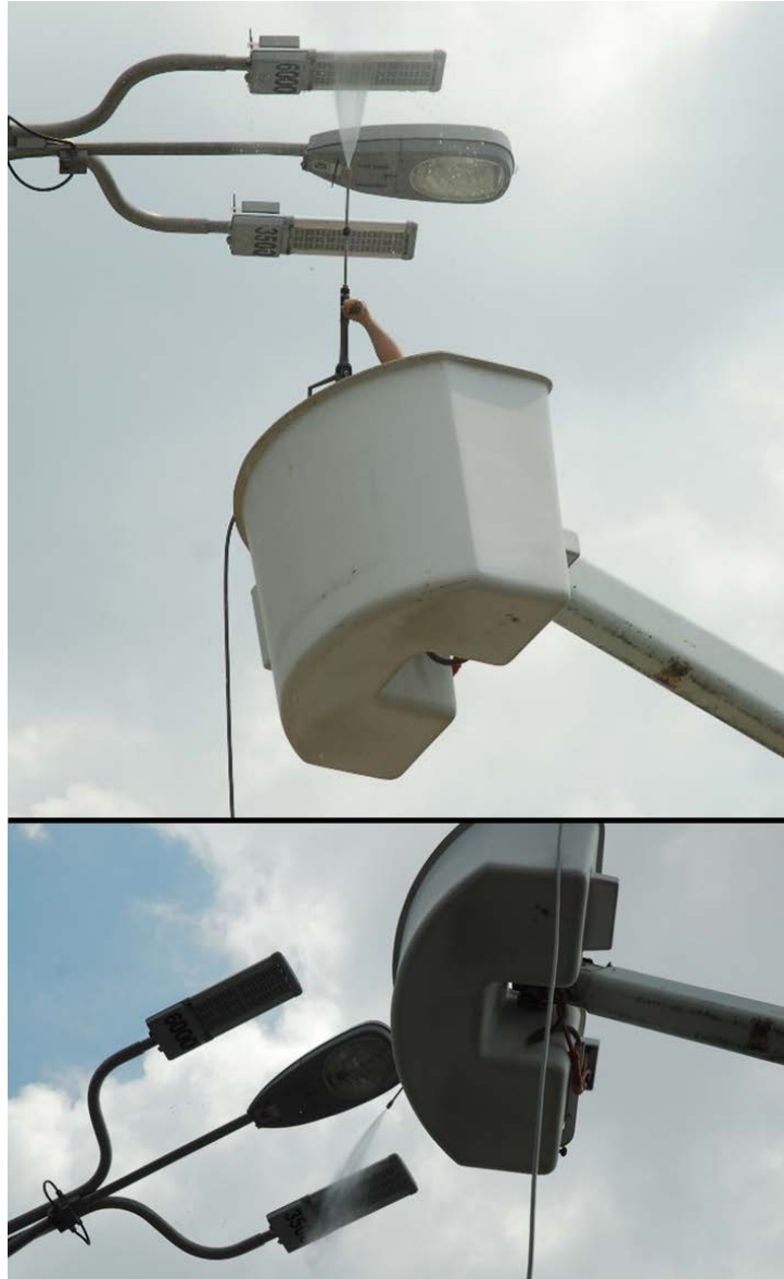
Figure 24. Pressure washing the optics of the Smart Road luminaires (Cleaning Method 4).
