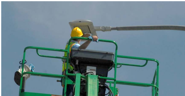
Figure 18. Cleaning an I-35W luminaire with IPA wipe.
