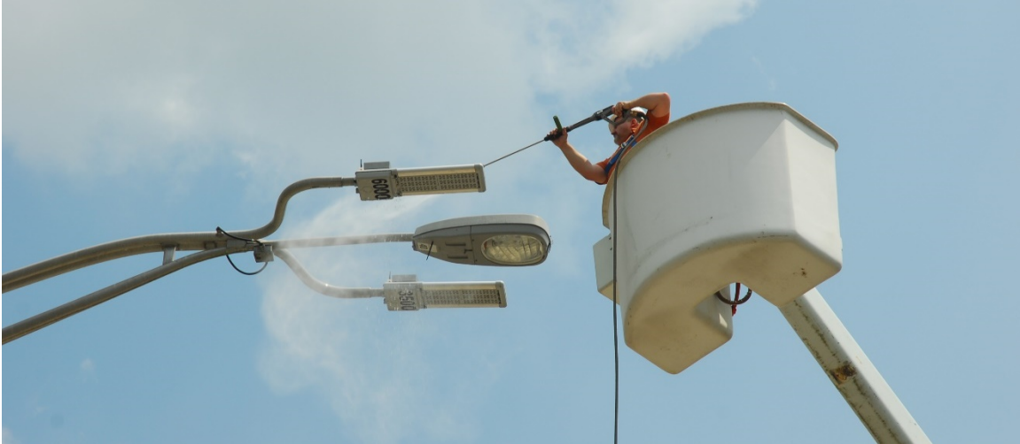
Figure 25. Pressure washing the heat sink of the luminaires (Cleaning Method 5).
