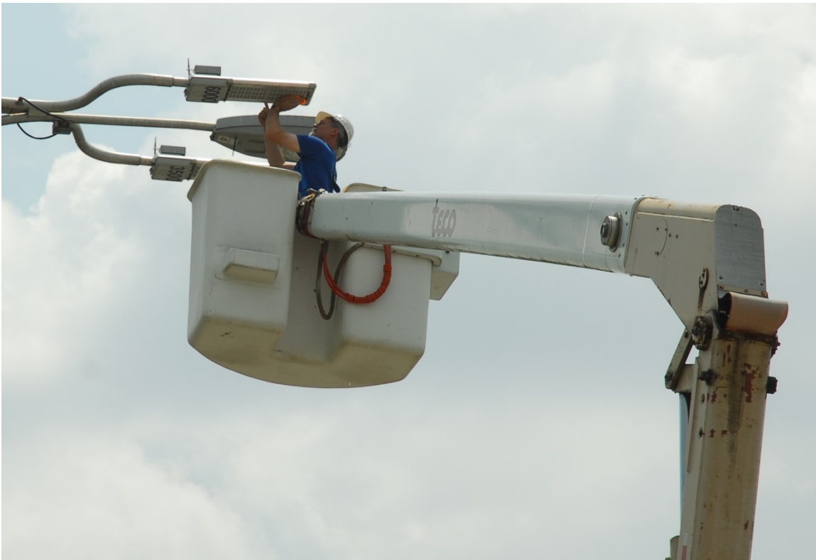
Figure 22. Wiping the Smart Road luminaires with a rag.
