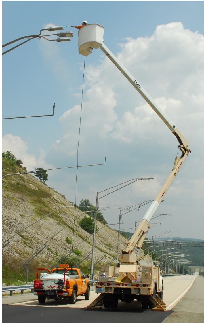
Figure 23. Setup to pressure wash luminaires on the Smart Road.
