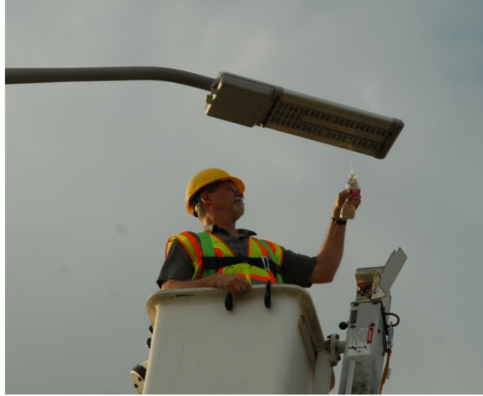
Figure 26. Cleaning a luminaire with water.
