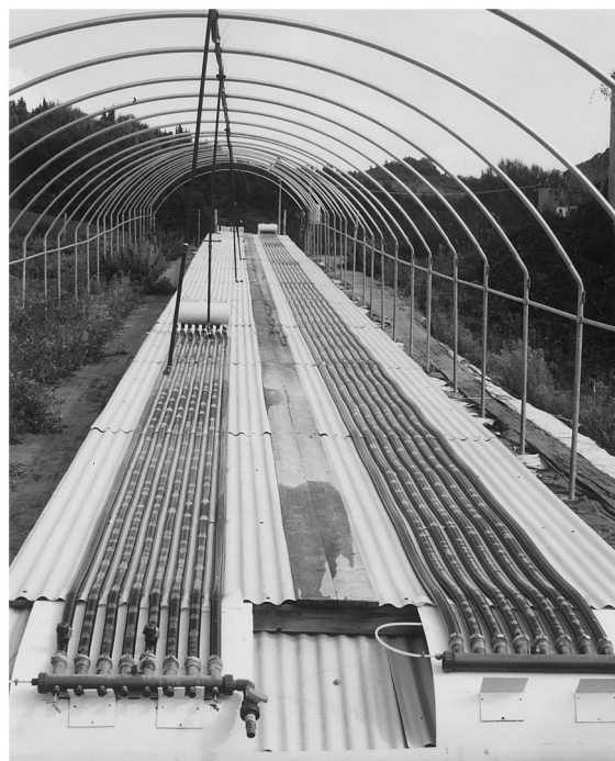
Fig. 1. Pilot eight-tube NHTR units installed at Azienda Agricola Montepaldi (San Casciano Val di Pesa, Florence, Italy).
